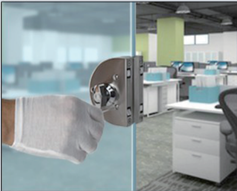
Step 3: Tighten the two short screws to secure the door lock(Almost enough)
