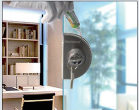
4 Step 4: Apply a circle of glass glue between the door lock and the glass for reinforcement
